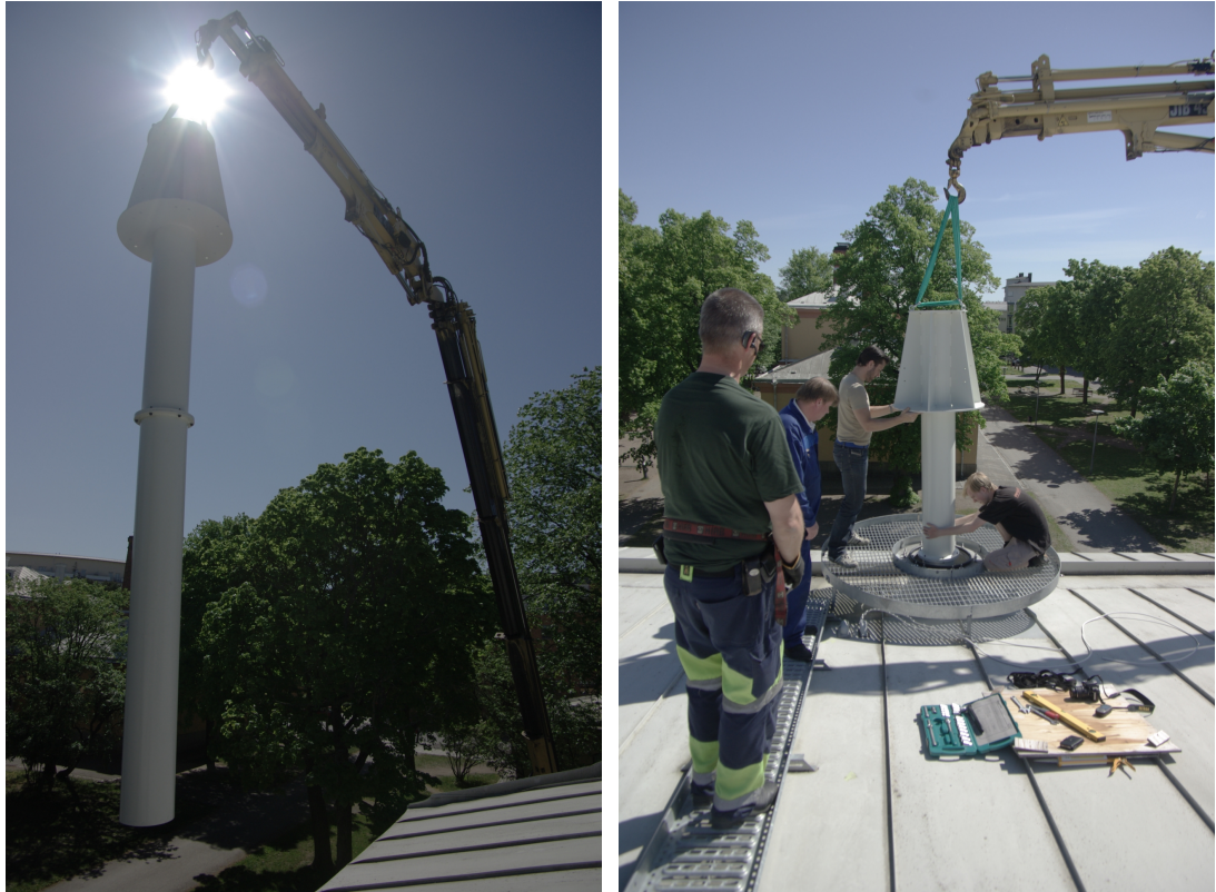
Figure 18: Lifting and mounting the beampipe
